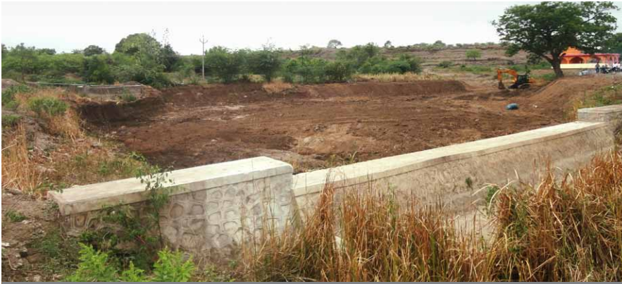
Renovation of Water Harvesting Structure
