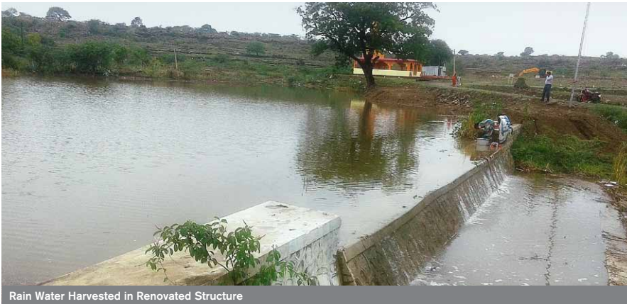
Rain Water Harvested in Renovated Structure
